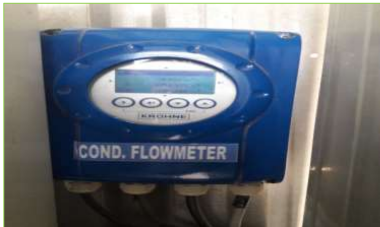
CONDENSATE FLOW METER IN ETP
