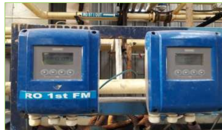
DOUBLE STAGE RO FLOW METER IN ETP
