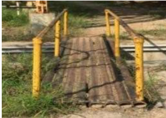
Ramps & supports made from scrap steel
