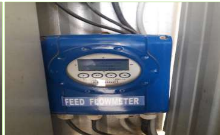
REJECT FLOW METER IN ETP
