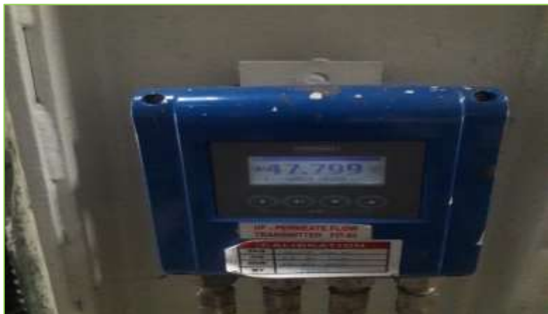
UF PRODUCT FLOW METER IN WTP
