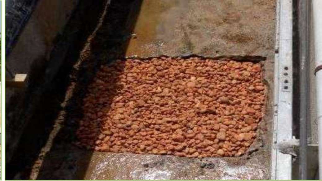
Percolation Pit in Drains – 30 Pits
