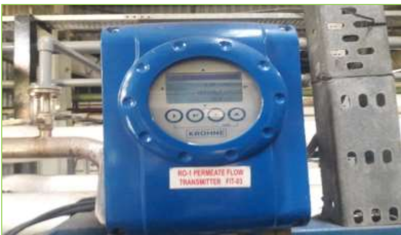
RO PRODUCT FLOW METER
